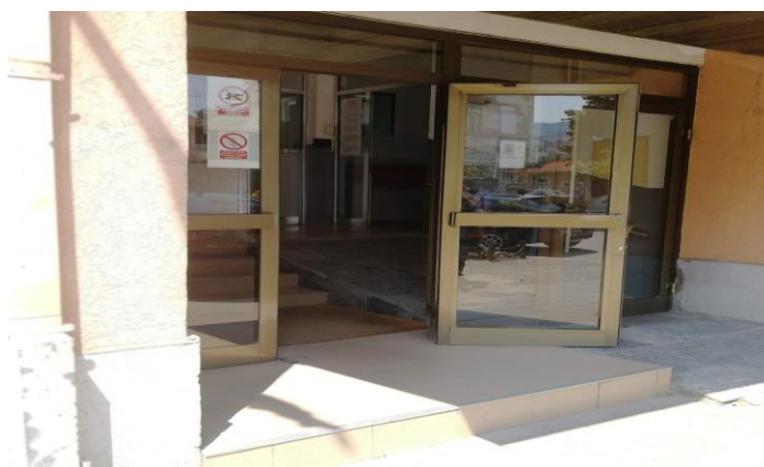
Image 4 – Lebane municipality, an example where the ramp on the right side of the entrance is steep and interrupted by closed doors
