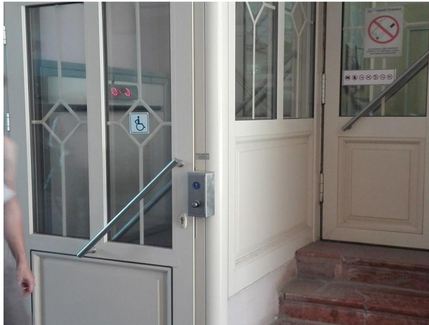
Image 1 – City house of Sombor: an example of the lifting platform which is user-friendly, safe and well fit into the architectural design of the space
