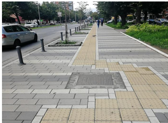
Image 6 – Tactile guiding line in Kraljevo where the panels used for tactile field of safety at pedestrian crossings are used to bypass the manhole which essentially is not even an obstacle to justify the increase of expenses (significantly greater number of tactile panels was placed than it was necessary) and it is repeated along the entire length of the street
