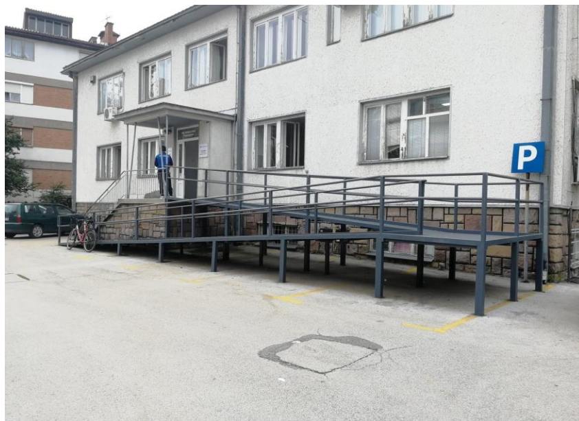
Image 13 – Health center in Pirot: Even though the ramp meets the standards (with the exception of the absence of a cover) and it is regularly maintained, it occupies four parking lots and the space is not used in the best possible way; it is necessary to find another solution which would occupy less space;
